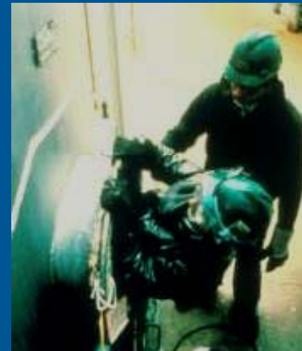
Confined space work
