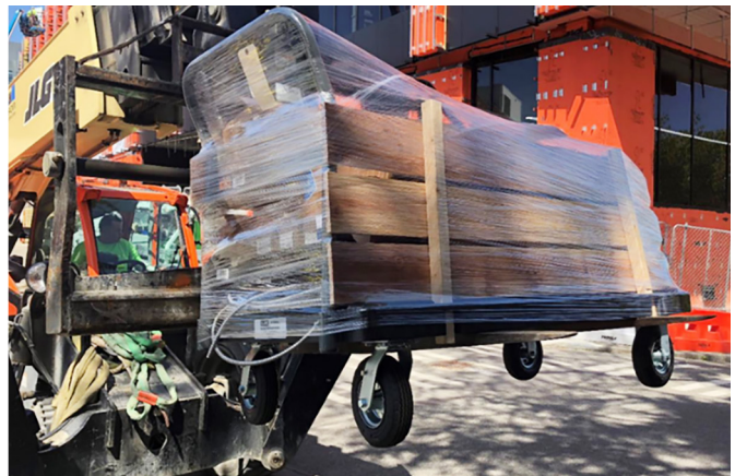
Fig. 1.3: Just In Time – Kitted Lighting Fixture Carts (Assembled off site, delivered on wheels, and taken to installation locations)
