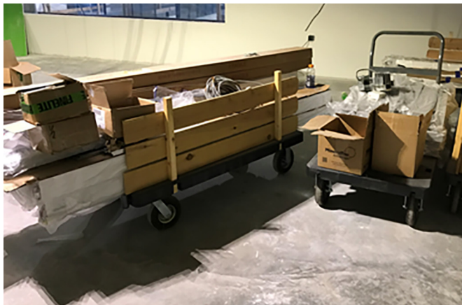
Fig. 1.3: Just In Time – Kitted Lighting Fixture Carts (Assembled off site, delivered on wheels, and taken to installation locations)
